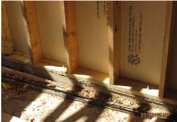
sill plate anchors
