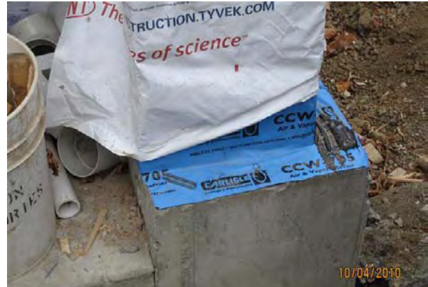
flashing @ masonry walls
