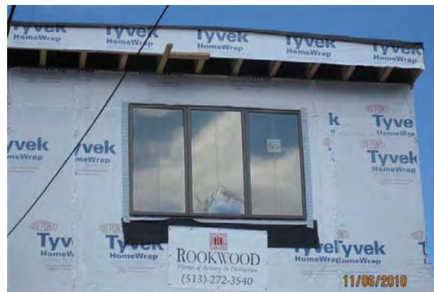
flashing membrane & tape @ openings
