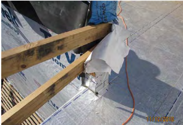
garage roof/deck flashing/counter flashing
