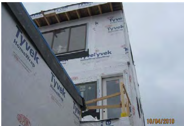
flashing membrane & tape @ openings
