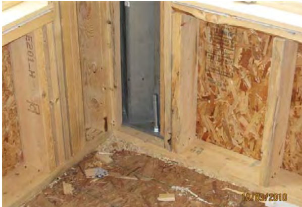
exterior wall cornering bracing, Simpson metal corner panels
