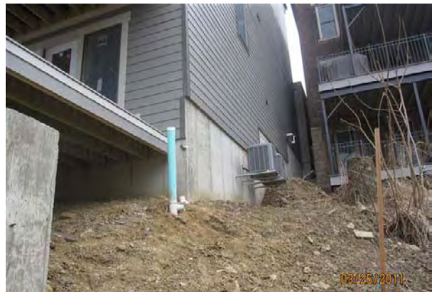
hold grade 8" below top of foundation
