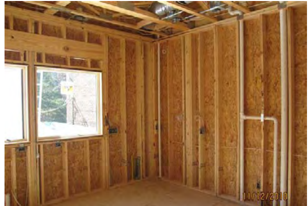
exterior wall corner bracing
