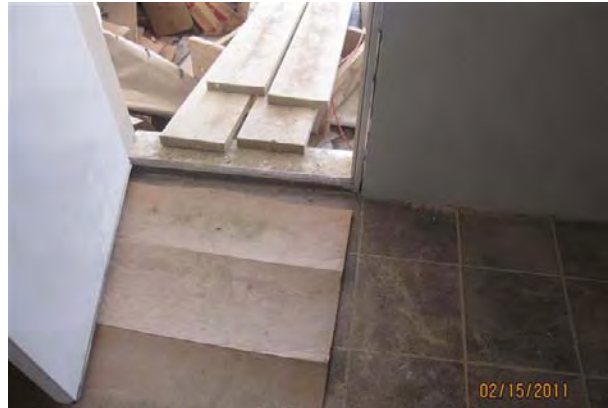
water-resistant flooring laundry room
