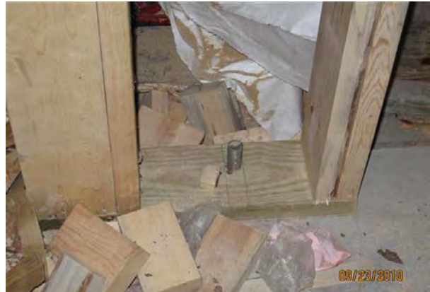
sill plate anchors
