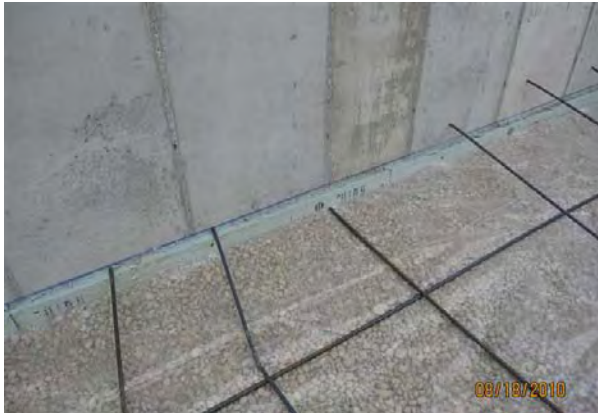
Under slab gravel, underslab vapor barrier
