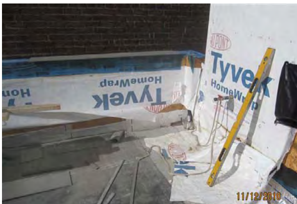
garage roof/deck flashing/counter flashing
