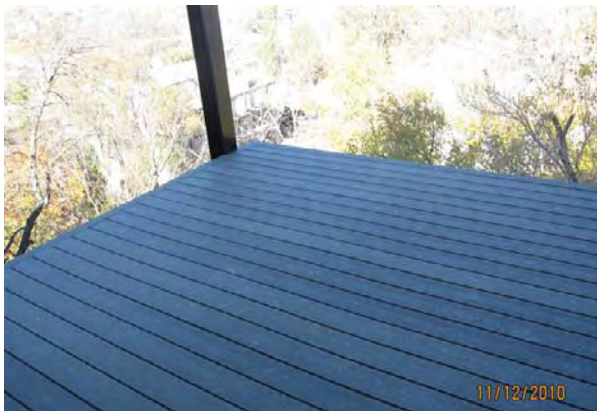
exterior hardiplank decking
