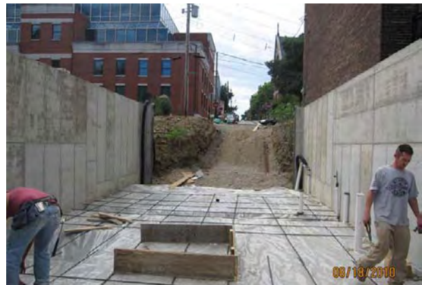
vapor retarder under slab, (2) interior foundation drains ready for pass thru @ South front wall @ garage
