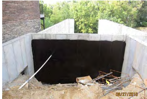
foundation damp proofing, underground downspout lines, gravel backfill
