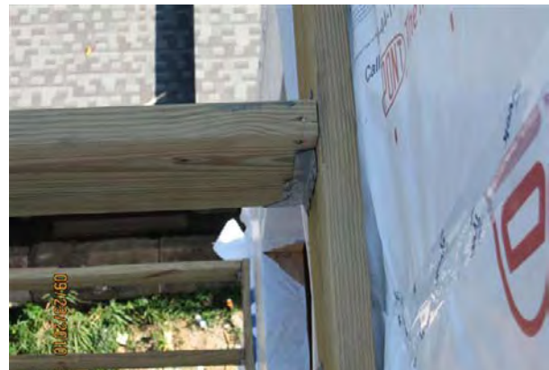
uninterrupted drainage plane @ ledger
