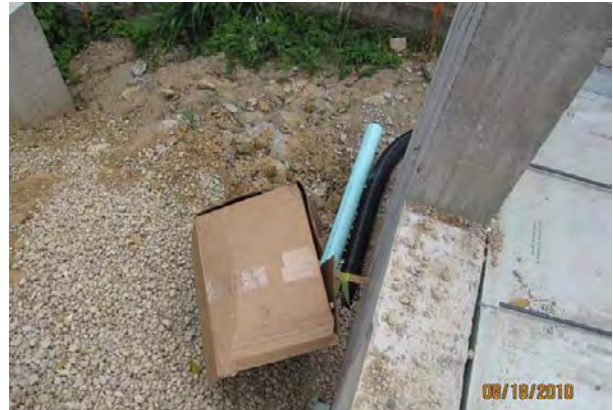
10" concrete foundation walls
