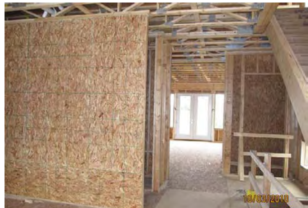
interior shear walls
