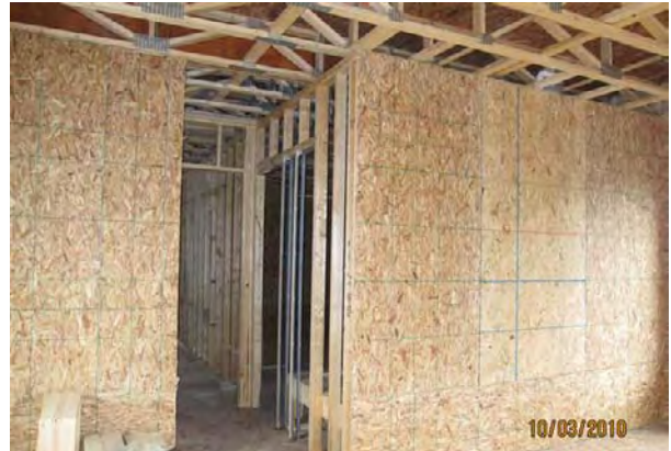
interior shear walls
