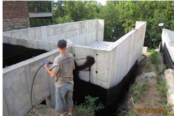
foundation damp proofing
