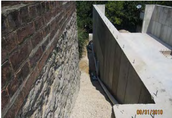
foundation damp proofing, underground downspout lines, gravel backfill
