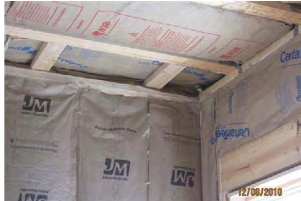
insulation over top plates
