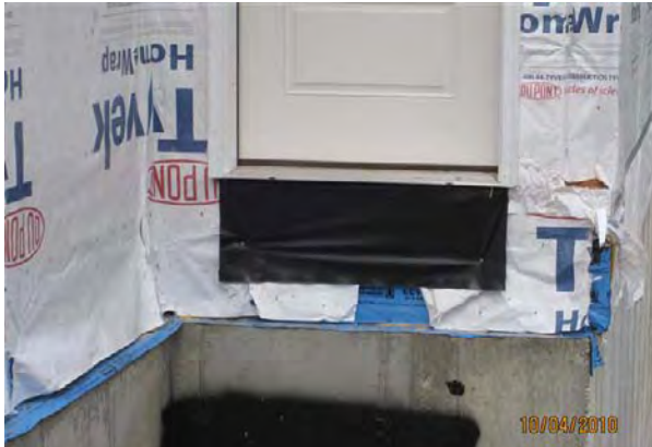
flashing @ masonry walls
