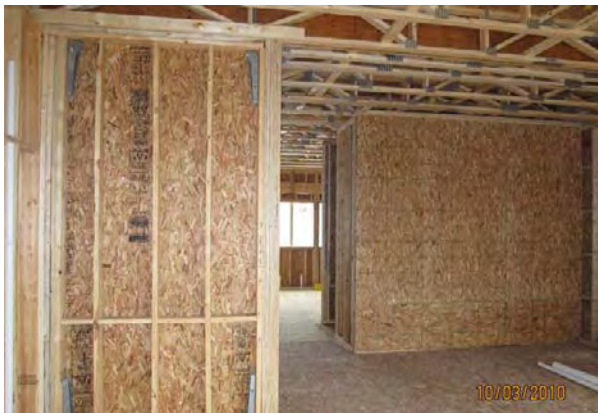
interior shear walls
