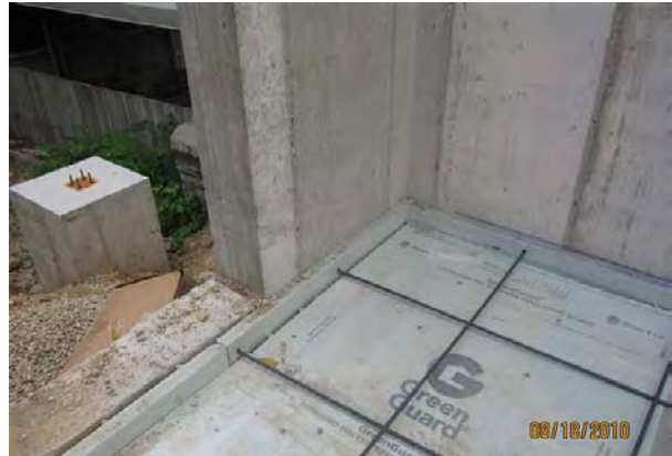
slab edge insulation @ walkout
