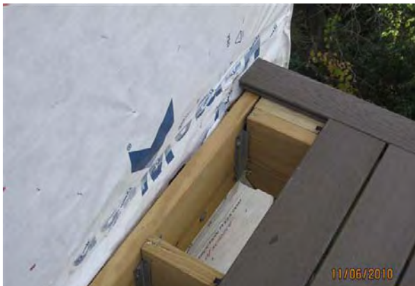
uninterrupted drainage plane @ ledger
