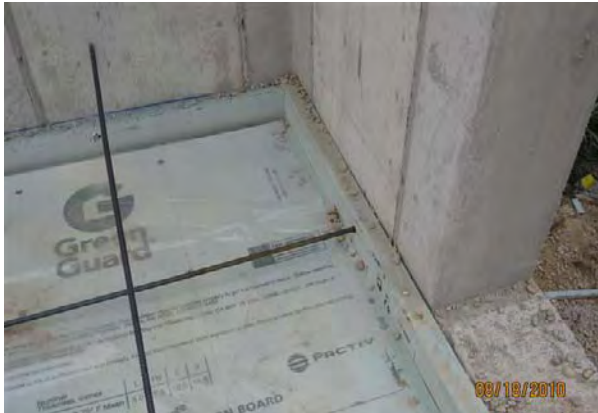
slab edge insulation @ walkout
