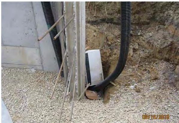
interior foundation drain thru rear exterior foundation wall, grade at North rear wall approx. 4' below lower level slab
