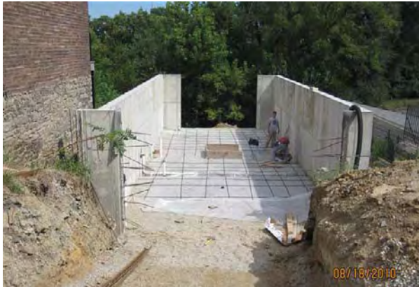
10" concrete foundation walls
