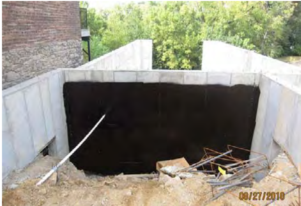
foundation damp proofing
