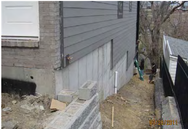
hold grade 8" below top of foundation
