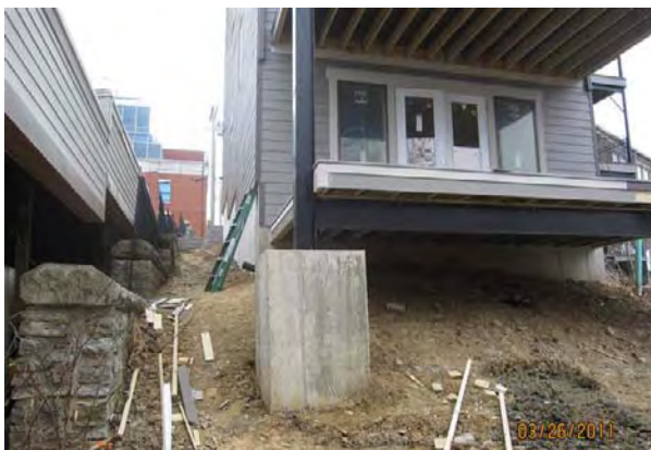
hold grade 8" below top of foundation
