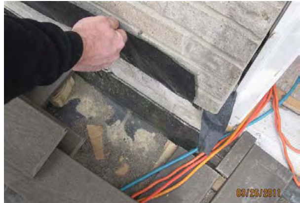
masonry flashing/counter flashing
